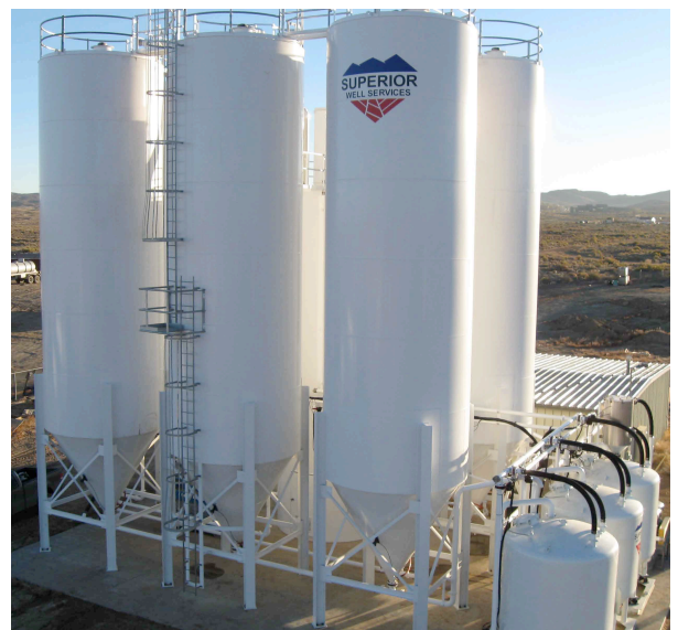
A Superior cement bulk plant.
